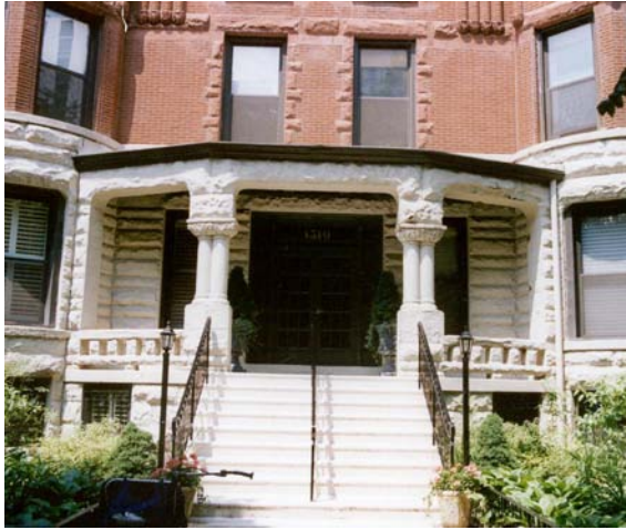
Before: Sandstone is painted, trapping water in the stone and obscuring the carved details.
