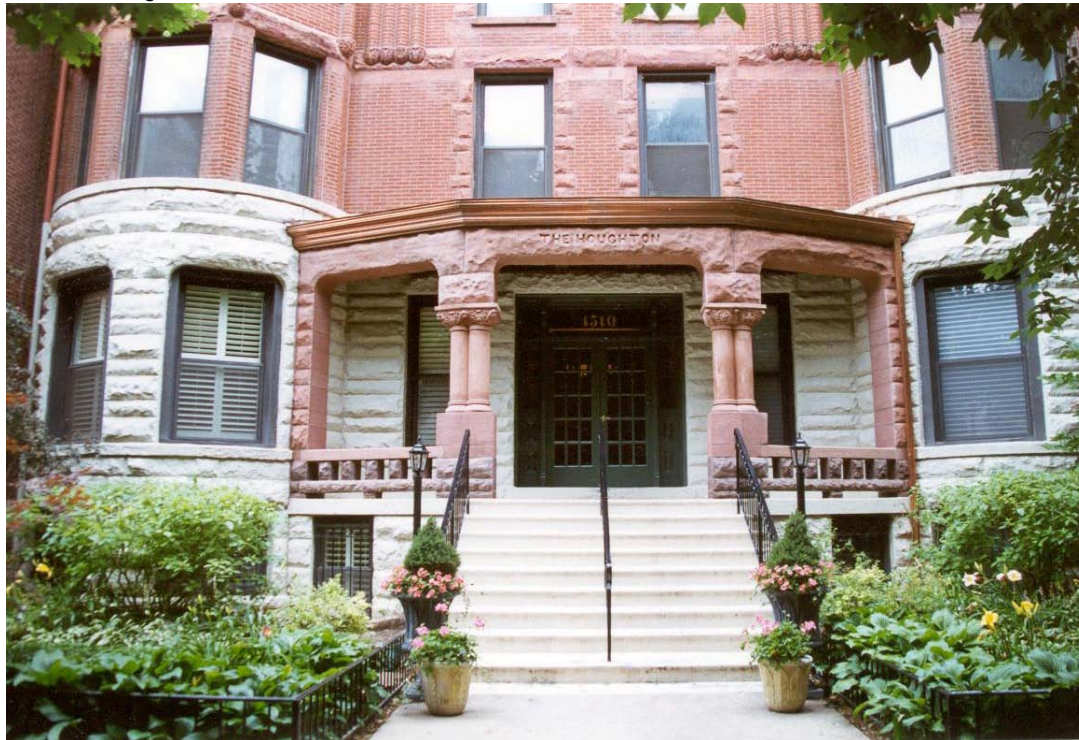
Before: Sandstone is painted, trapping water in the stone and obscuring the carved details.
