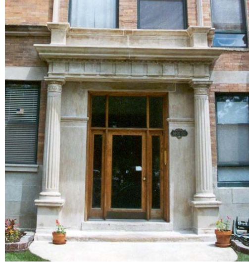
Fig. 2 After. The stone was patched to restore it to its original appearance and repointed. Patching material – Heritage Limestone Restoration Mortar HL15
