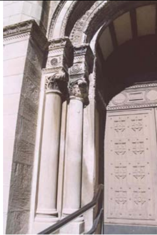
Fig 2. Capital in the portico selected for sample stone repair.
