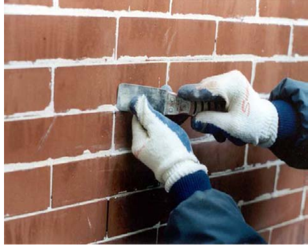
Fig 2. To ensure that the brick is not damaged when the mortar is removed, it is necessary to find the joint. In the most sensitive manner possible, gently scrape off the mortar adhered to the face of the brick.
