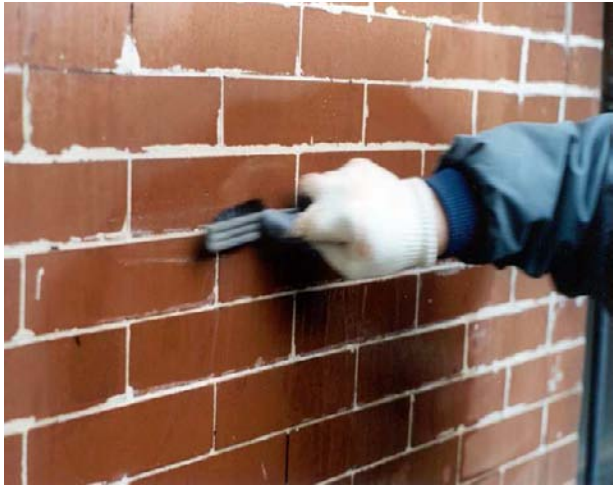
Fig 4. Scrub away the stains and mortar residue using a brush with nylon or natural bristles.
