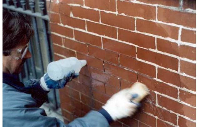
Fig 10. Once all mortar has been removed from the joints, wash away dust and particles with water and a brush. This helps in two ways: It prevents replacement mortar adhering to masonry, it also prevents shrinkage crack formation (the brick will not absorb water from the mortar). Before installing material, eliminate standing water.
