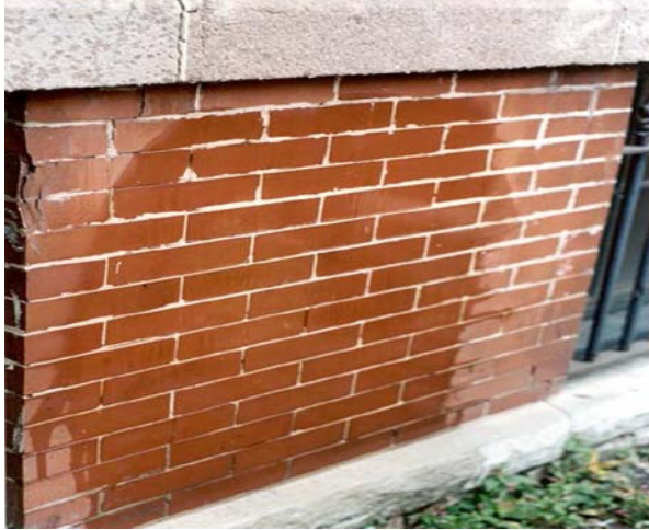
Fig 5. Thoroughly saturate the wall with water; by doing so, the lime present in the original mortar is softened, making the mortar easier to remove.
