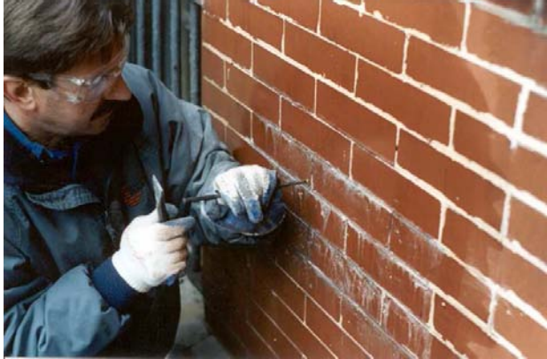
Fig 9. After the center of the mortar joint has been cut, use hand tools to carefully remove mortar from the sides of the brick.
