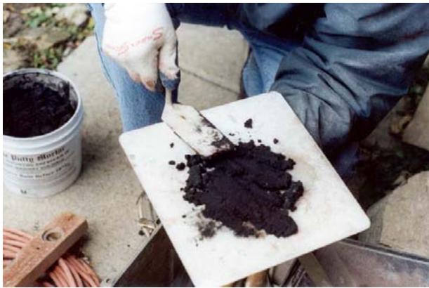
Fig 11. Load your hawk with a relatively dry and stiff mortar mix. A sufficiently dry mix will compact well and prevent shrinkage cracks.
